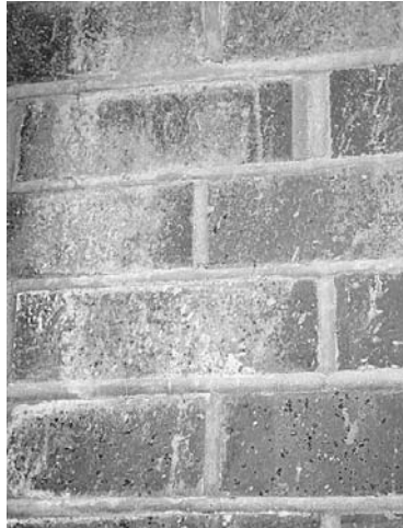
Figure 16-2 Efflorescence.
